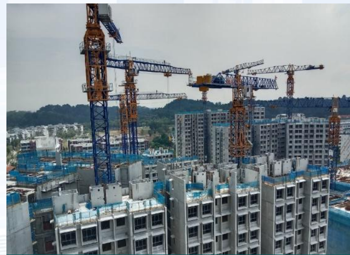
LẮP DỰNG (ASSEMBLY)
